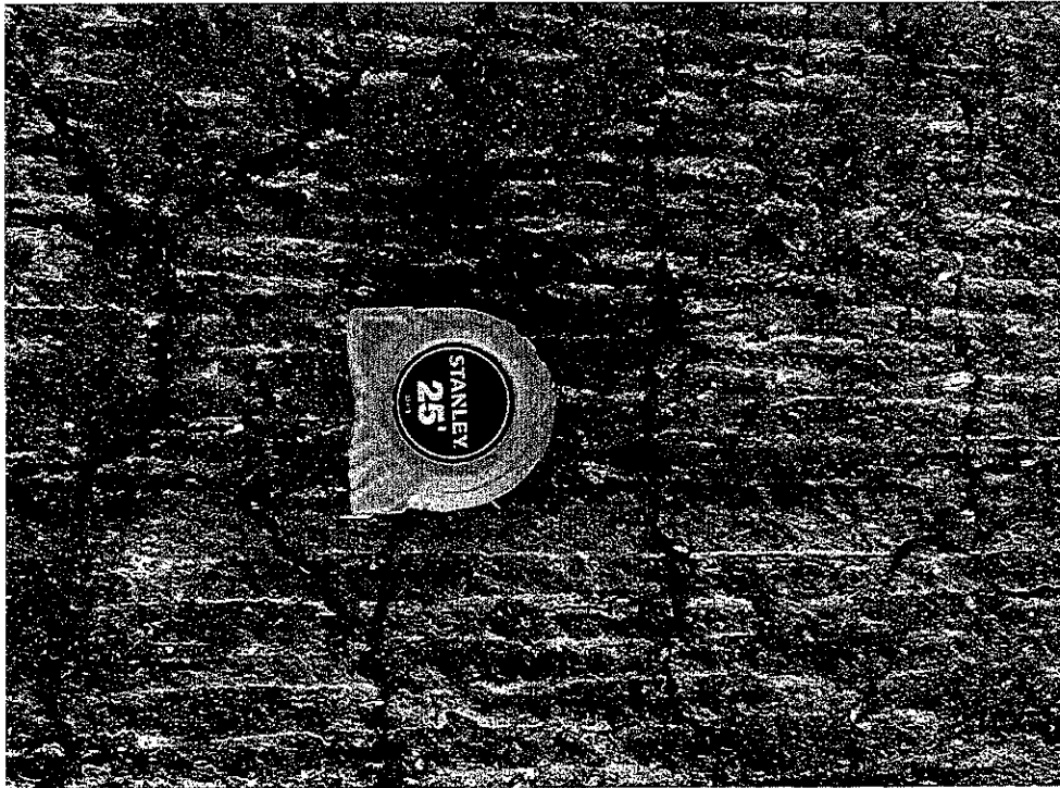
Microcracking of milled runway surface associated with brittle asphalt.
